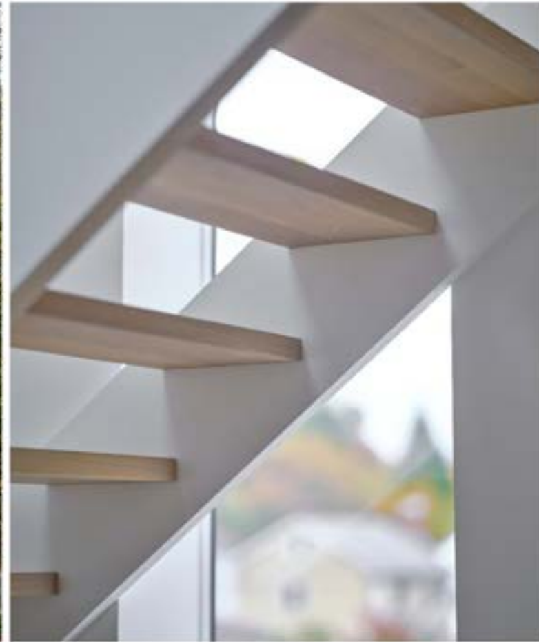
Fig. 18. Close-up view of modern staircase opening within existing
