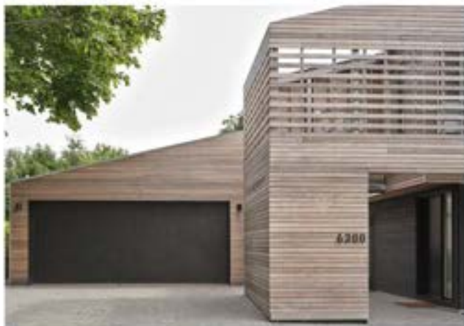
MAIN ENTRY, OUTDOOR WOOD STORAGE AND SCREEN
