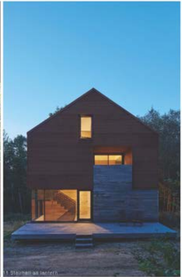
11 Stairwell as lantern
