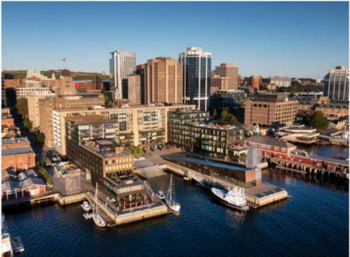
2 Development comprises three abstracted ships set perpendicular to and supporting a 330 ft. sandstone "bar" building.
