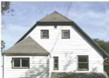
Figure 5. Existing structure restored to original and exterior stone stone house light.
