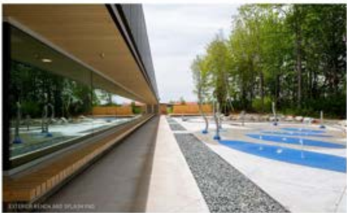
EXTERIOR DECK AND SPLASH PAD
